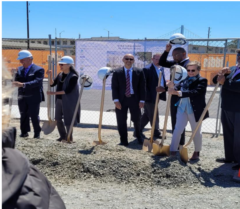
Figure 2 Groundbreaking event for Treasure Island Star view Court
